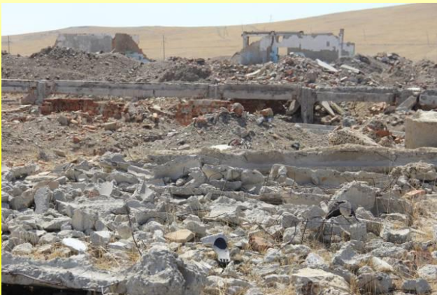
The ruin of old heating plant in Bayantumen
