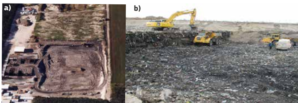
From left to right: a) Aerial view of the site at the beginning of the clear-up operations b) Excavation of municipal waste with a skeleton-excavator
