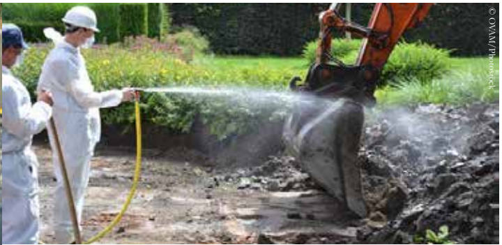
Belgium. Large-scale asbestos remediation works
