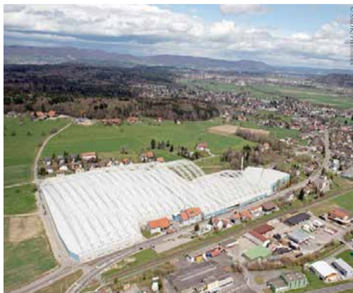
The site of the Kölliken hazardous waste landfill showing complete enclosure for the remediation works (2007- 2018)
