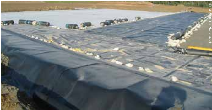
Belgium, Bois Saint-Jean. Remediation works
