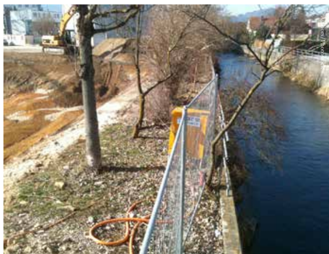
On the left, the polluted site of the former gas plant, on the right, the nearby river "Sorane"
