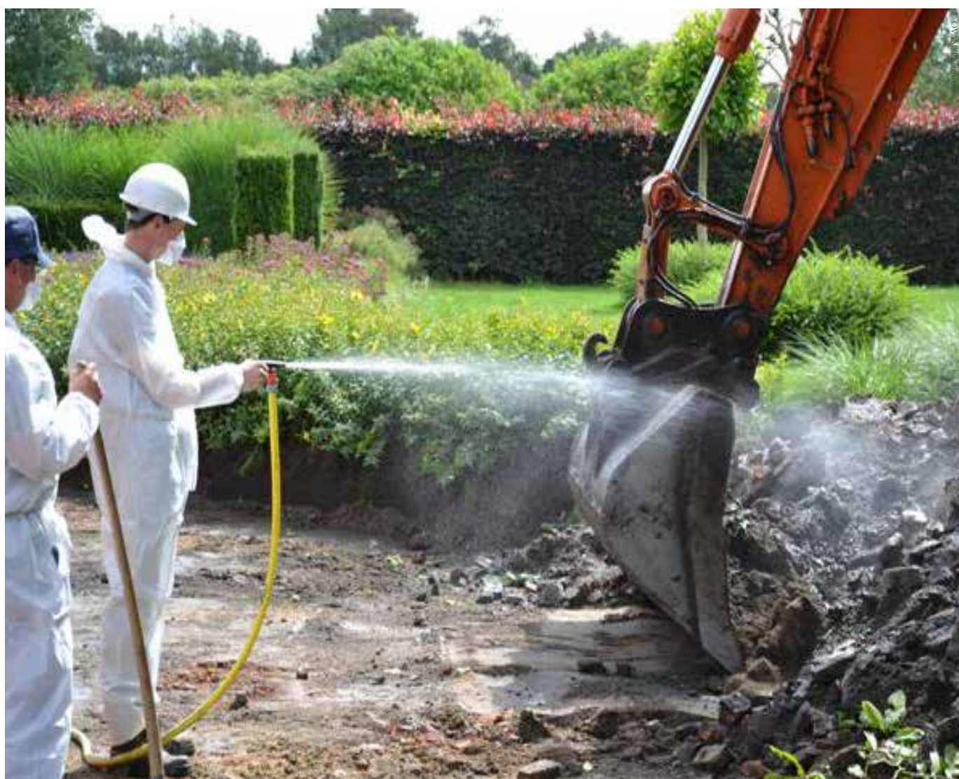
Workers removing asbestos
