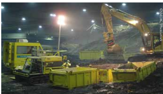
Typical configuration of the landfill dismantling activities during the first dismantling stage (2007-2009).
